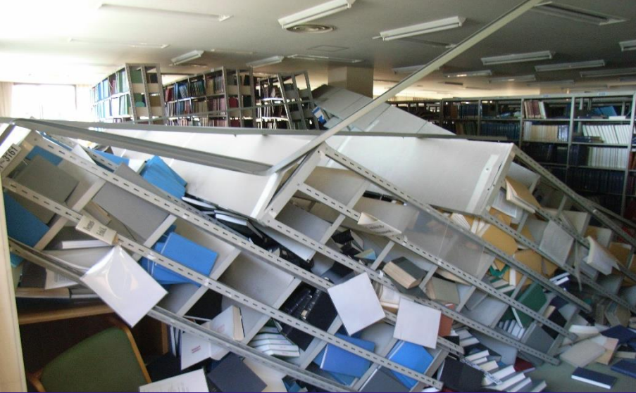
Bookshelves collapsed while being connected
